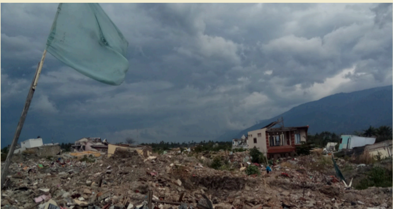
Figure 2. Post-earthquake and liquefaction conditions in Central Sulawesi
